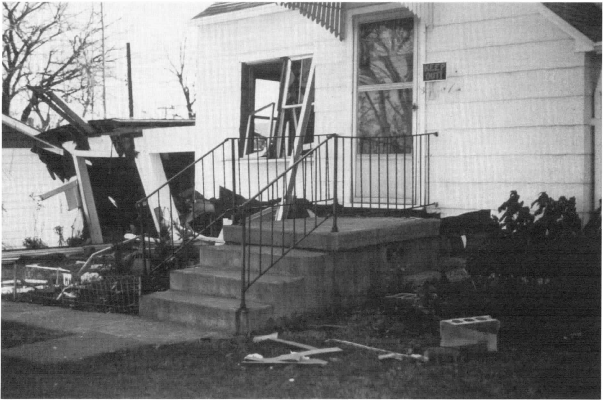
Figure 13-3.1 Low order damage in a dwelling.
