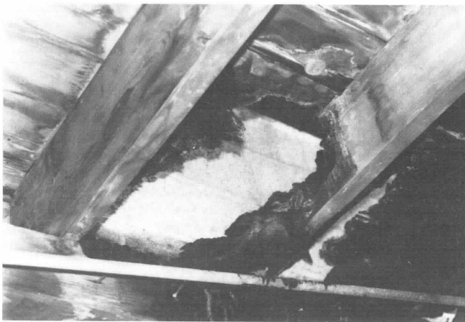
Figure 4-17.10 Saddle burn in a floor joist.
