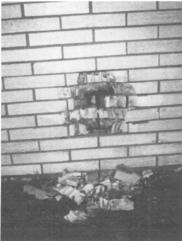
Figure 4-20.2 Damage to an outside brick wall caused by thermal expansion of an I-beam in the basement.
