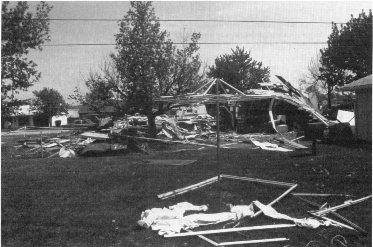
Figure 13-3.2 High order damage shown by shattered and splintered remains of a four-bedroom house.
