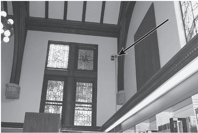
FIGURE F.4(c) Linear Beam Smoke Detector.
