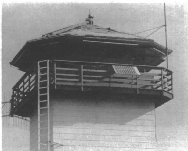
Solar collector panel on mountaintop lookout.
