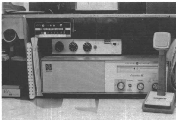
Portable base station with public address system, an 8-frequency scanner at top as installed in fire station.
