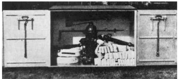
FIGURE A.4.2.5.3(a) Hose House of Compact Dimensions for Installation over a Yard Hydrant. Construction can be steel or aluminum.
