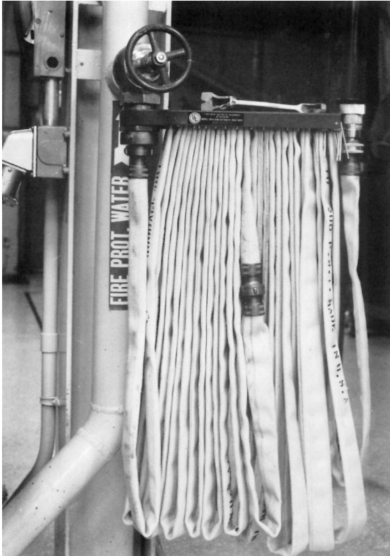
FIGURE A.4.3 Typical Standpipe and Fire Hose Rack Arrangement. (Courtesy of National Aeronautics and Space Administration.)
