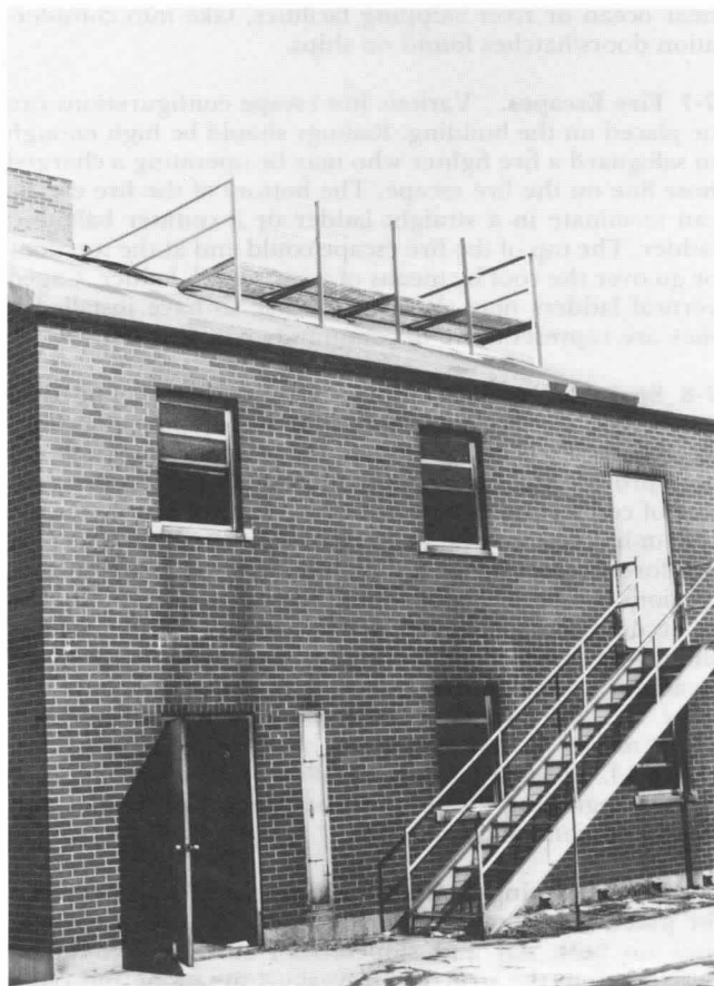
Figure 7-9 Safety railing roof of smoke building. Burlington County Fire Academy, Burlington County, New Jersey.
