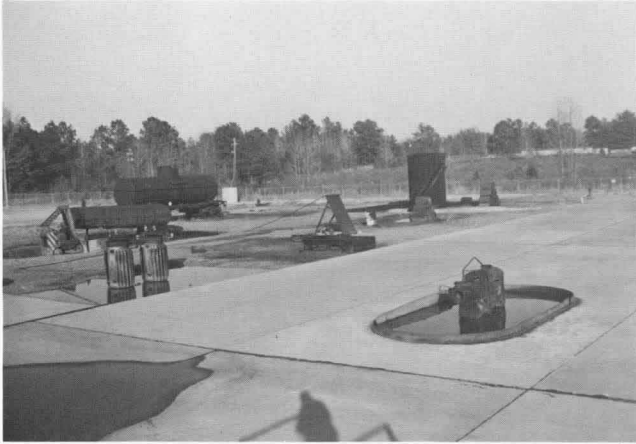
Figure 11-2 Flammable liquid burn area. Area includes cross pit, oval pit, square pit, electrical transformers, baffled pit, running spill area, drum pit, vertical tank, horizontal tank, and railroad tank car. Mississippi Fire Academy.
