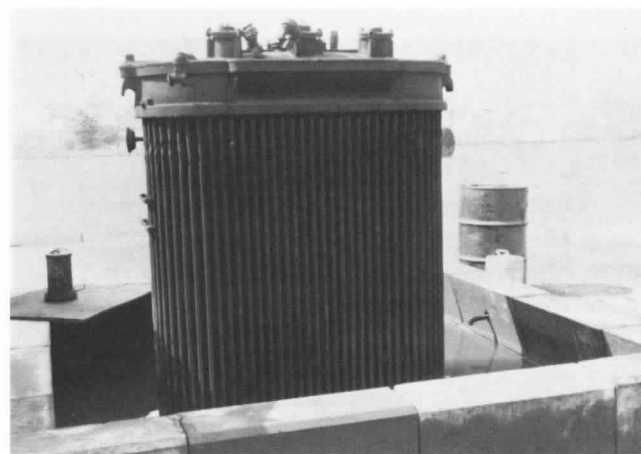
Figure 11-2.3(f) Flammable liquid cooled electric transformer mock-up. Note diking to contain runoff.
