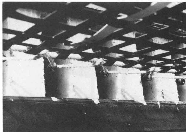
Figure 7-11(b) Springs anchored into the side of the drill tower. New York Fire Department Fire Academy, New York, New York.
