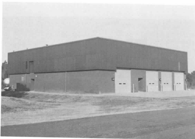
Figure 10-1.2(a) Fire apparatus building classroom. This building is approximately 100 ft (29.9 m) long with five 15-ft (450-cm) over-head doors, classroom, maintenance area, and apparatus storage area. Mississippi Fire Academy.
