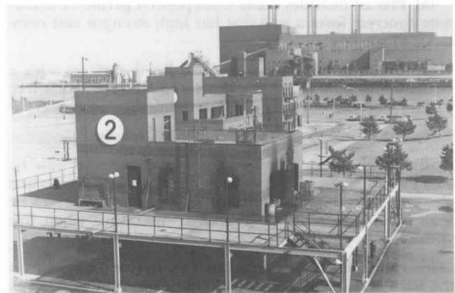
Figure 8-1.1 Burn building with raised open grid walkways level with the second floor. New York Fire Department Fire Academy, New York, New York.
