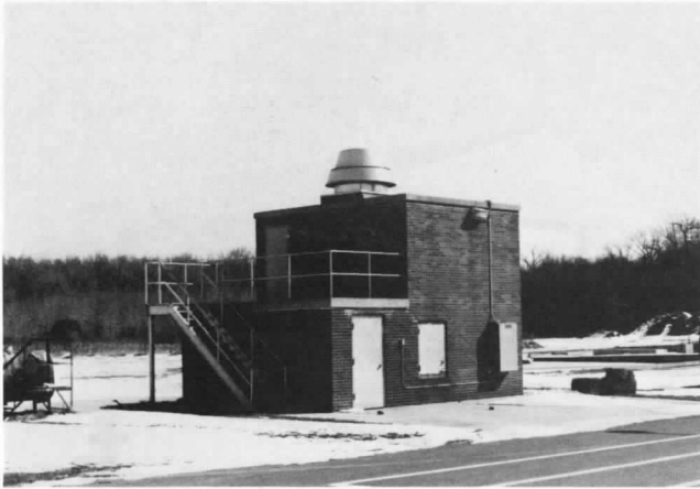
Figure 9-1.1 Smoke building with exhaust fan at roof level. Burlington County Fire Academy, Burlington County, New Jersey.
