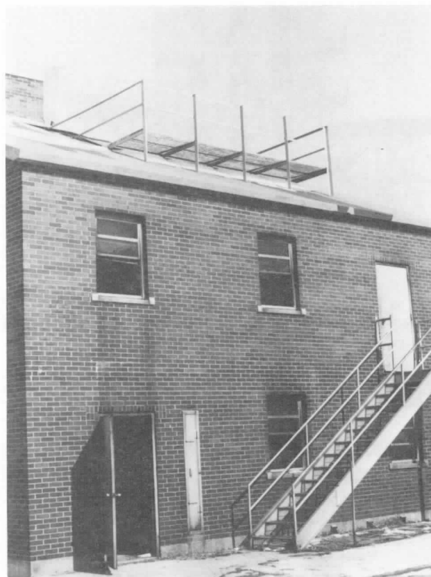
Figure 7-9.1 Safety railing roof of smoke building. Burlington County Fire Academy, Burlington County, New Jersey.
