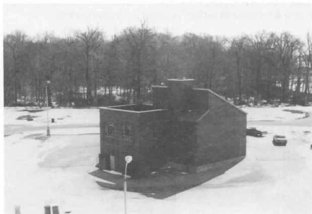
Figure 8-1(b) Burn building consisting of a private dwelling section and a commercial section. Burlington County Fire Academy, Burlington County, New Jersey.
