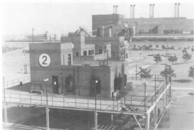
Figure 8-1.1 Burn building with raised open grid walkway level with the second floor. New York Fire Department Fire Academy, New York, New York.
