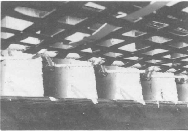
Figure 7-11.1(b) Springs anchored into the side of the drill tower. New York Fire Department Fire Academy, New York, New York.
