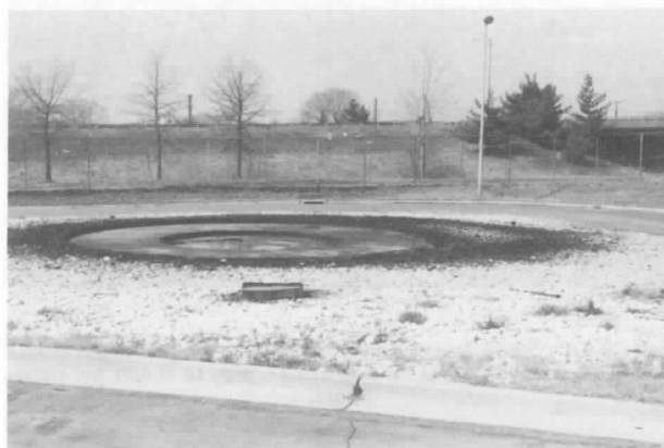
Figure 11-2.2 District of Columbia Fire Department flammable liquid pond. Note heavy stone surrounding pond.
