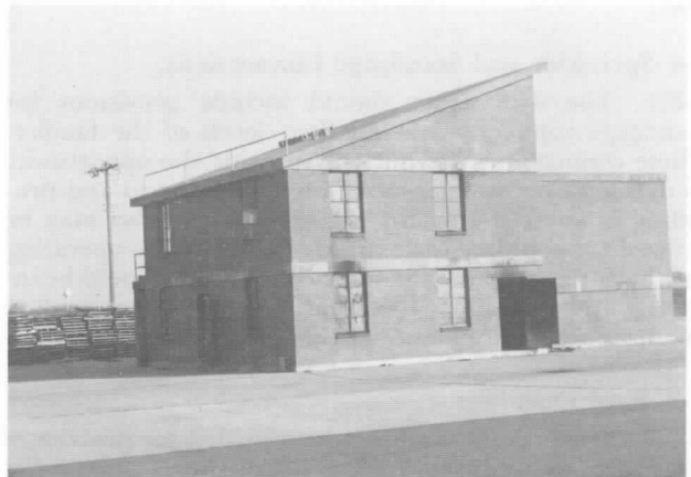
Figure 8-1(a) Hot drill building. This building features two buildings in one — residential and commercial. The residential side is two stories with attic, six interior rooms, all masonry. Mississippi Fire Academy.
