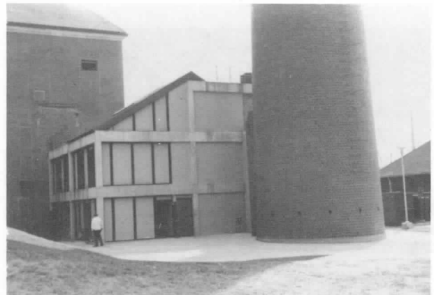
Figure 10-1(b) Combination building — maximum use of minimum space with existing smoke stack for EPA considerations. Building provides for ventilation; smoke chamber; rappelling; ladder; live fire training; sprinkler laboratory; gas and electric cutoff; and forcible entry.
