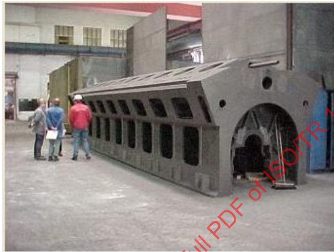
Figure 29 — Large cylinder block to be repair welded
